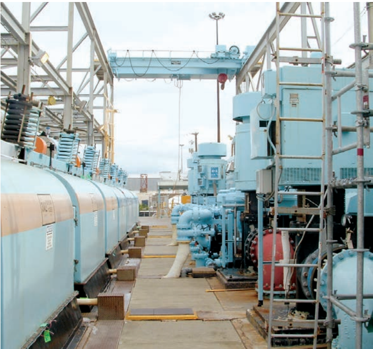
The above-grade portion of existing traveling water screens (on the left) must be removed and replaced by the new MultiDisc Screens to protect the pumps (on the right) from debris. Photo/Site
