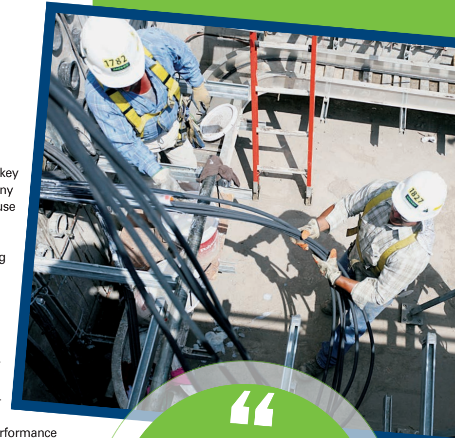
Electricians Alvaro Lara (left) and Jose Sierra (right) pull cable in an electrical manhole. Photo/Alissa Hollimon
