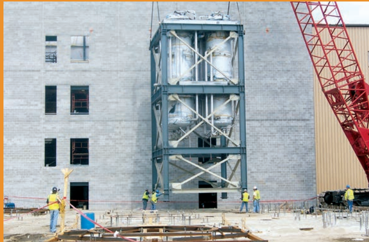
The first of 24 modules is set on a foundation prepared at the site. The seed fermenter makes up part of the interior structure and working floors of the building.
