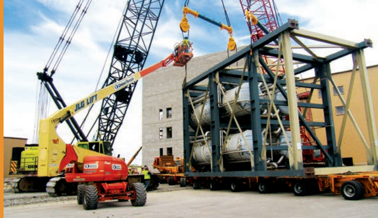
The seed fermenter arrives on the site and is rigged to be lifted into place. Once the module is removed from the heavy-haul trailer, it will be turned upright and ready to be placed on the foundation.
