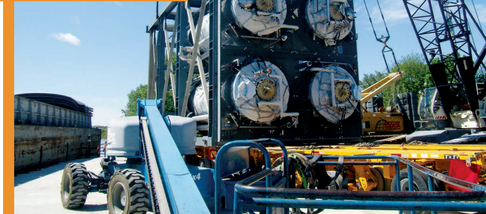
A seed fermenter, fabricated in China, gets offloaded from a barge on the Missouri River and set onto a heavy-haul trailer to be transported to the site. Zachry also designed the river unloading station used here. Photos/Site
