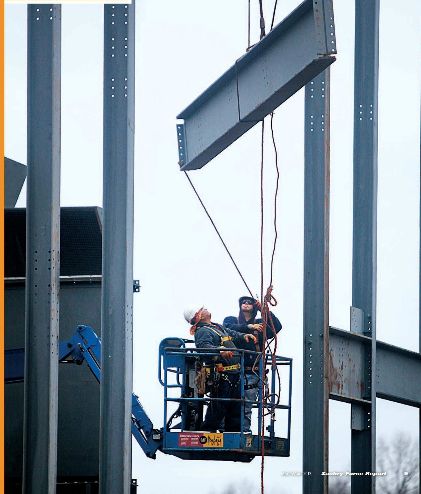
David Howard and Freddie Garcia, both structural ironworkers, work from a lift basket to guide a piece of steel into the air pre-heater/economizer structure.
