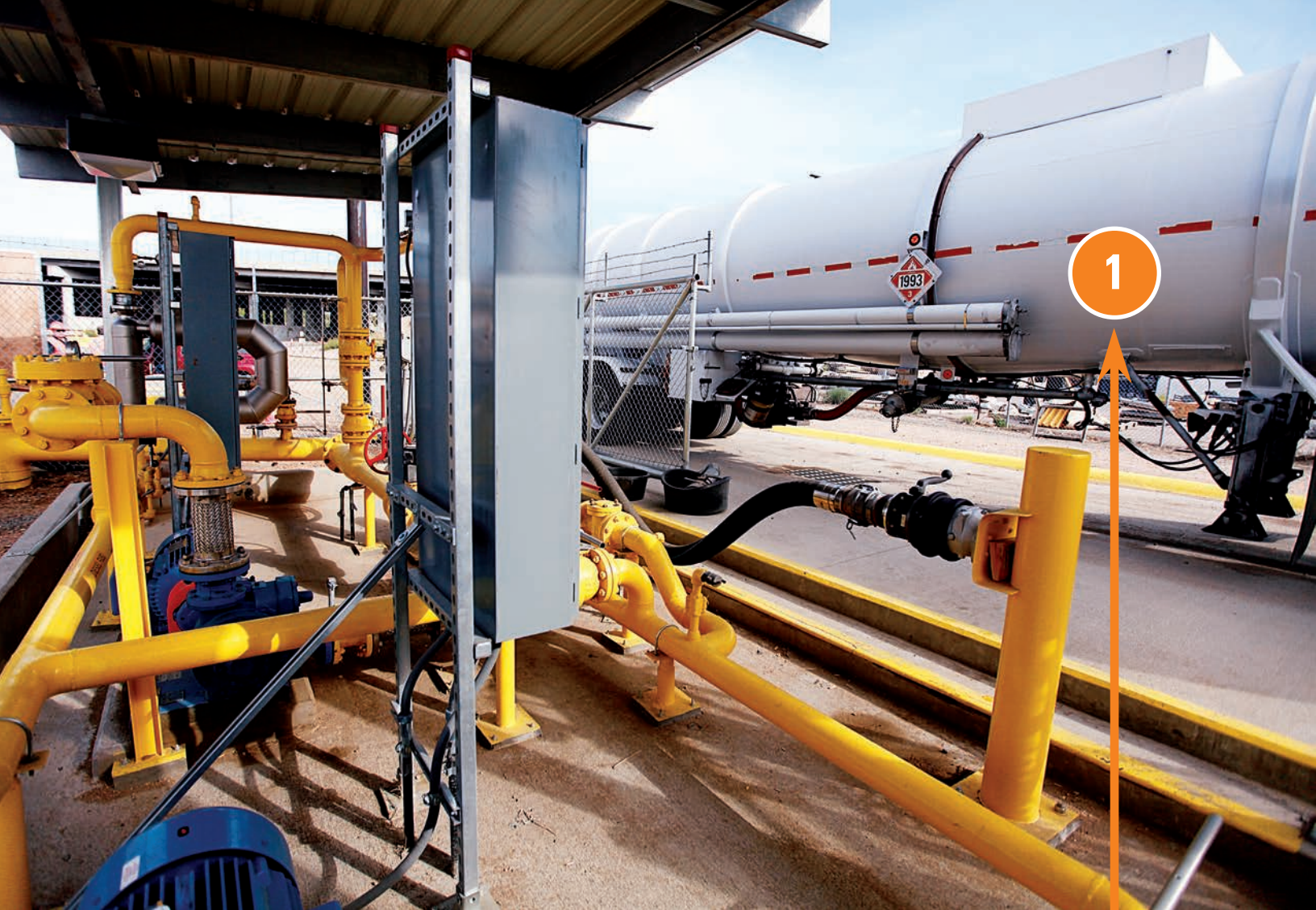
The diesel fuel oil (DFO) truck loading and unloading system at the Globeville Rail Yard in Denver, Col. Photos/Alissa Hollimon
