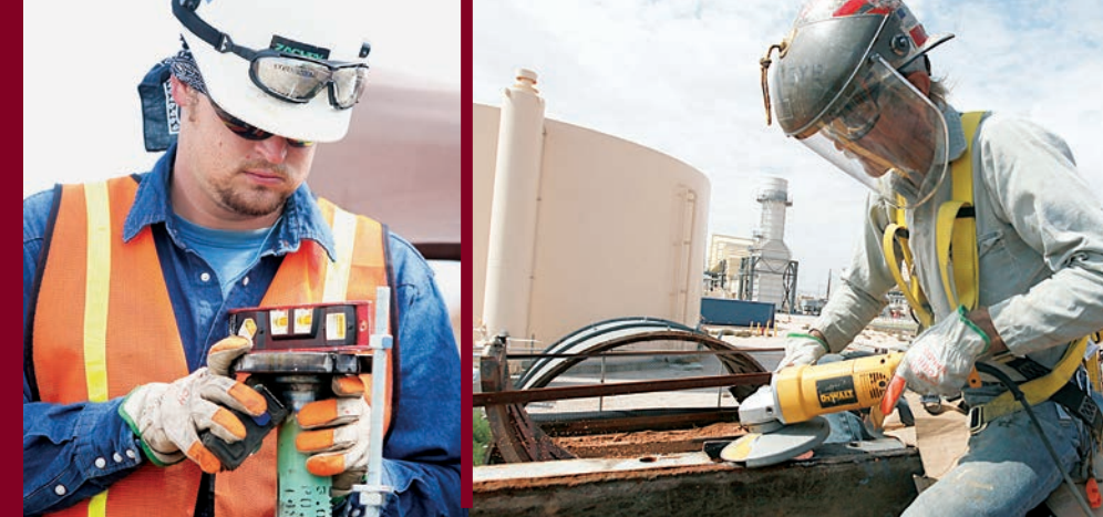
(Left) Pipefitter Chris McClain checks the level of the top of a pipe that will be embedded under the combustion turbine. (Right) Structural Ironworker Jay Krout grinds slag on the exhaust stack. Photos/Alissa Hollimon
